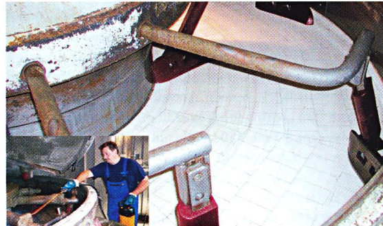
Fig. 2 The application of the mixing cleaning agent is quite simple.
